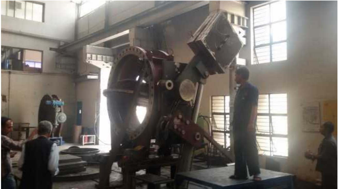
Inspection of valve
