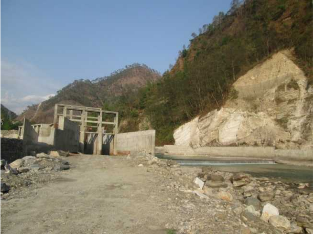
Headworks from downstream
