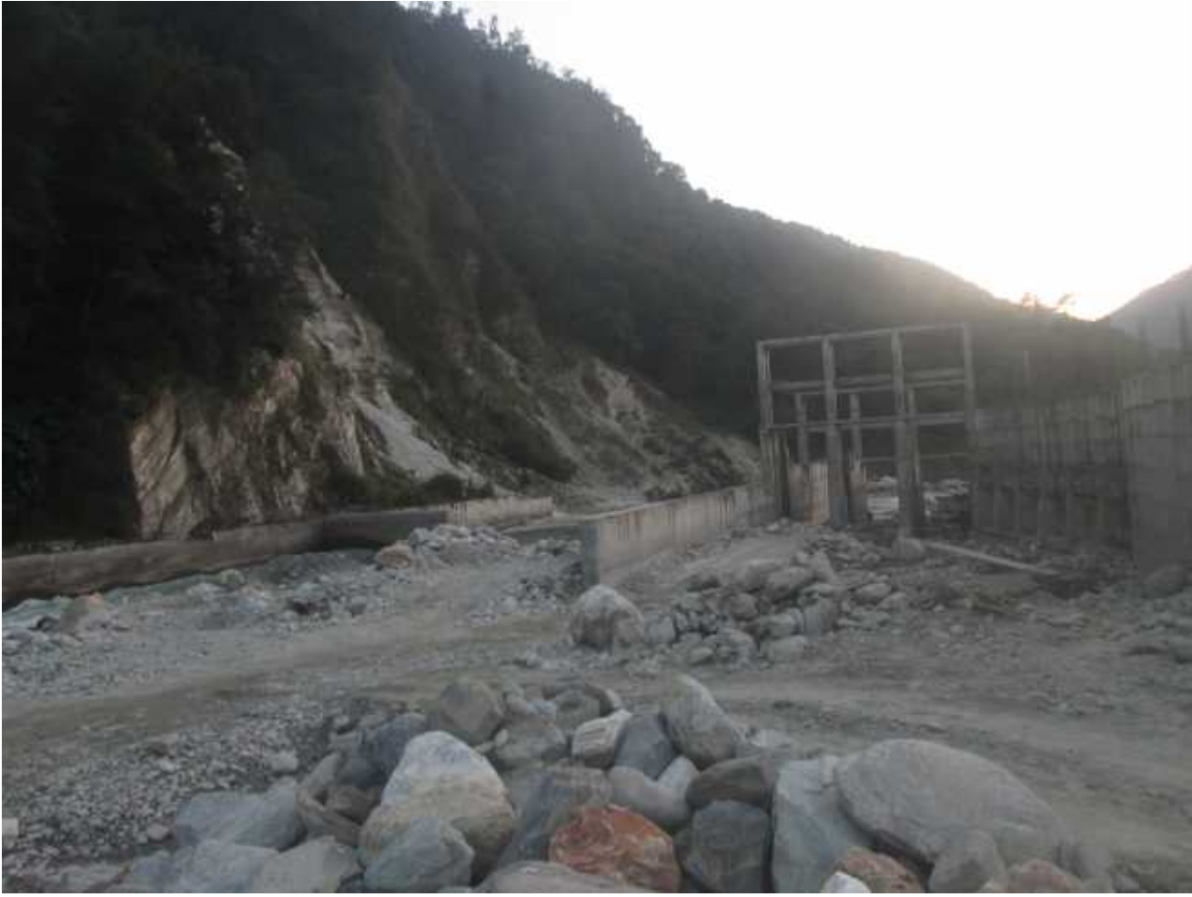
Headworks from upstream
